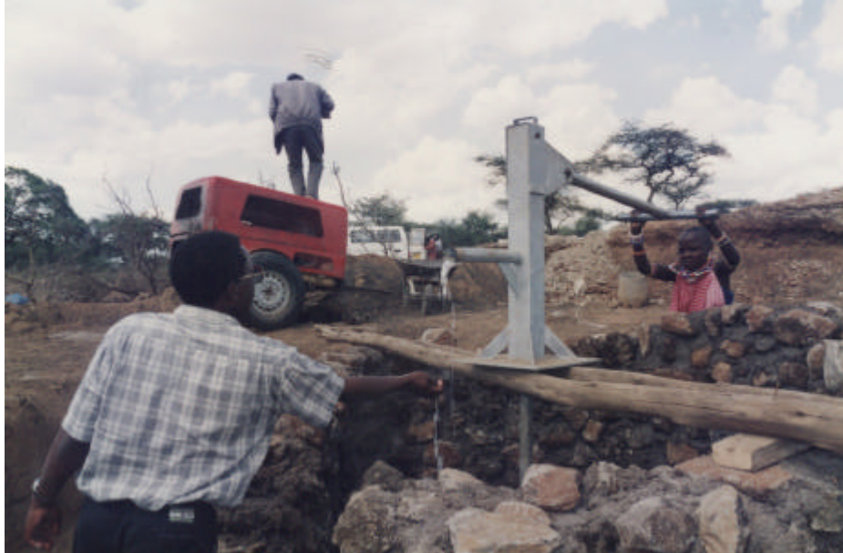
Figure 8: Placing and testing a hand pump
